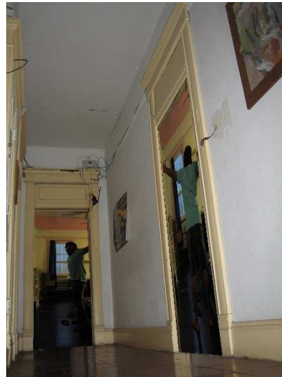
(e) Another example of the open doors warped to the doors.
